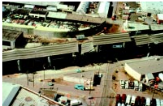
Collapse of Interstate 880 from the 1989 Loma Prieta Earthquake that killed 67 people and caused an estimated 7 billion dollars in property damage, much of that to the transportation system. (NOAA)
